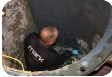
Sea water filter was in need of urgent repair. The internal surfaces were abrasive blast cleaned and lined with 2 coats of 202 Ceramic Repair Fluid. The coating was then post cured at 50C for 6 hrs to ensure the filter was back in operation within 24 hrs.
