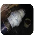
Leaking pipe sockets on a diesel pipeline at a European oil refinery wrapped and sealed using 104 Metal Repair Fluid XF
