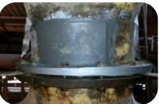
Emergency repair to seal a leaking flange face on a cooler box
