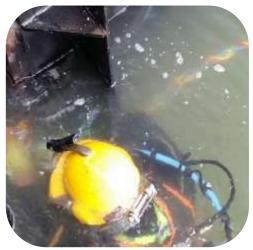
Seal and rebuild damaged or worn surfaces underwater. 106 Metal Repair Paste XF can cure underwater at temperatures as low as 5° C
