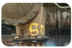
Cold bond steel plate to seal leaking pipe surfaces
