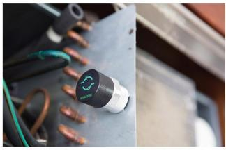
Wireless vibration sensor mounted on panel
